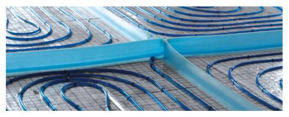
Fig. 14. Distribution of heating fields with dilatation gaps
